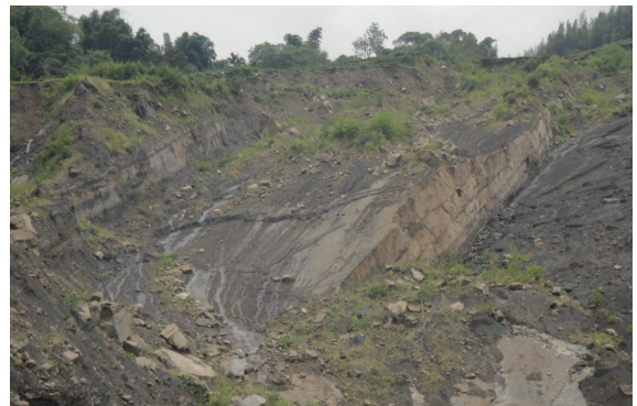
圖 10 G 區崩場地照片，滑動面主要受層面控制 Fig.10 Photo of the area G. the slide plane is controlling by bedding plane
